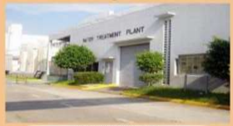
INSIDE THE WATER TREATMENT PLANT
